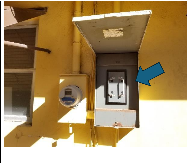
Pull-Out Fuse Main Disconnect Panel
