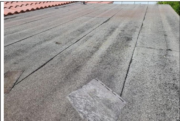
Missing Granules / Old Roof (see next photo)
